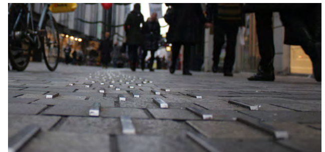
Aural/'noise' paving: integrated 'rumble strips' provide an aural warning cue for approaching traffic at intersections and turns. NO SOURCE FOUND
